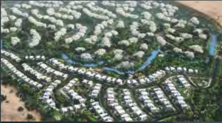
The Nest (99 villas), Wadi Al Safa, Dubai, U.A.E. Client: Al Barari Development Co. Consultant: Emkaan Engineering Consultancy Main Contractor: Sustainable Builder (Al Barari Development)
