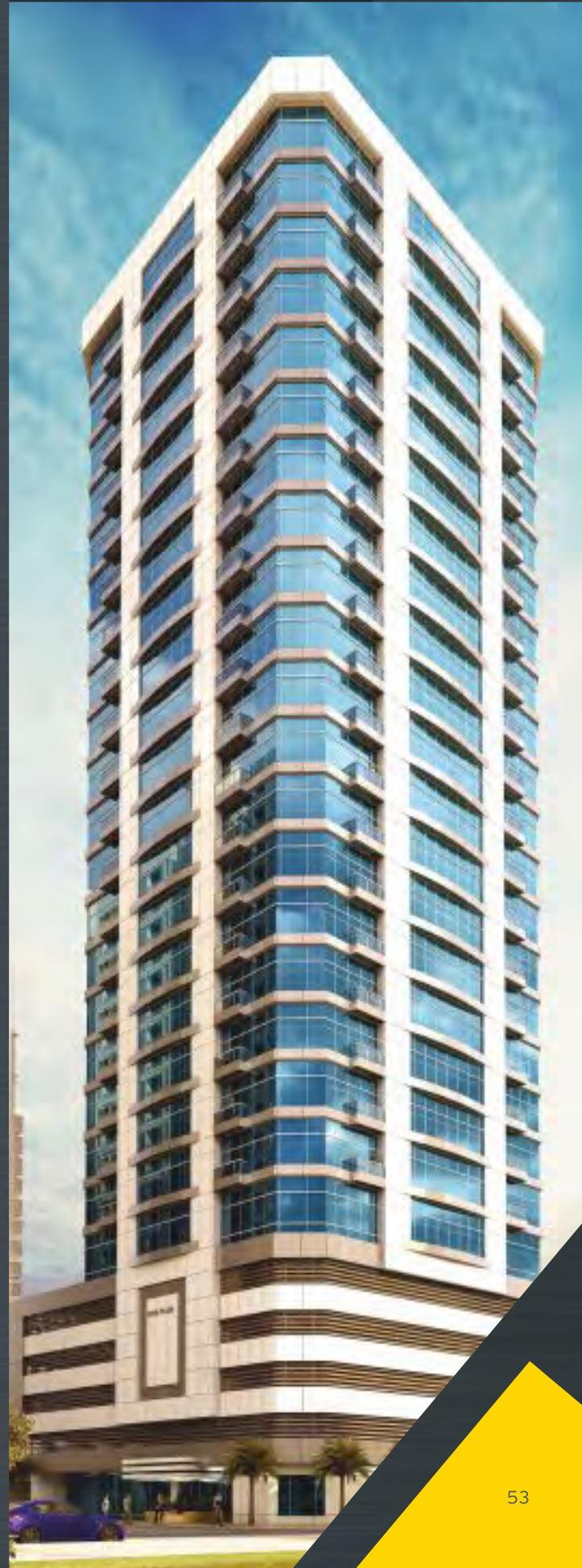
Suha Plaza Project , Manama, Bahrain Client: Suha Investment Consultant: Aref Sadeq Design Consultants Main Contractor: Juma Construction
