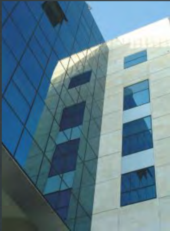
Tadrous Building Commercial Complex Amman, Jordan
