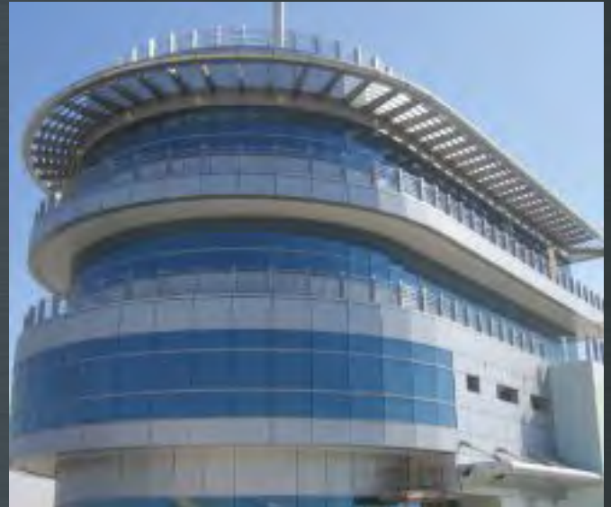
Dubai Maritime City - Control Building Dubai, U.A.E.
